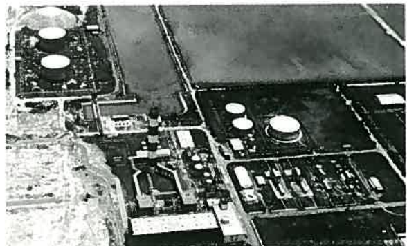
GRESIK STEAM POWER PLANT (PLN,INDONESIA)
