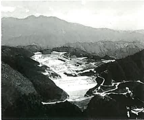
KURIYAMA DAM (TEPCO, JAPAN)
