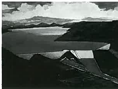
Bili-Bili Multipurpose Dam Project, South Sulawesi, Indonesia
