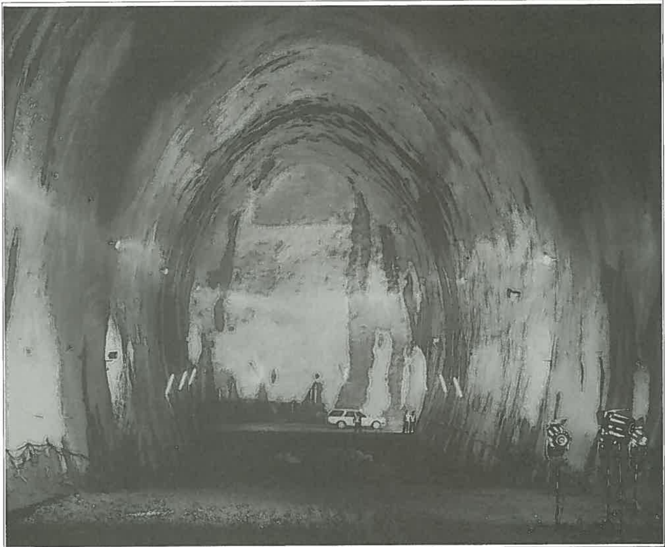
Kuji Underground Crude Oil Storage Tank
