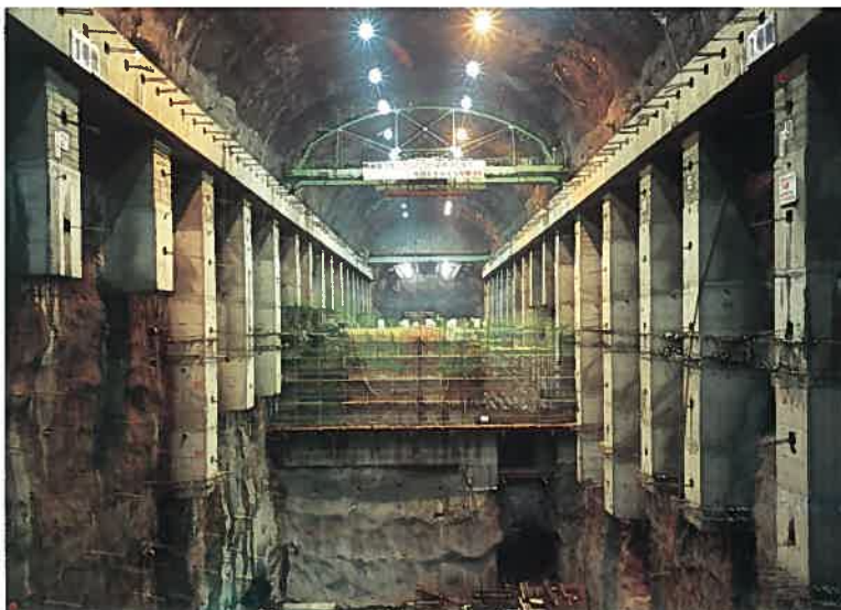
Okawachi Power Station
