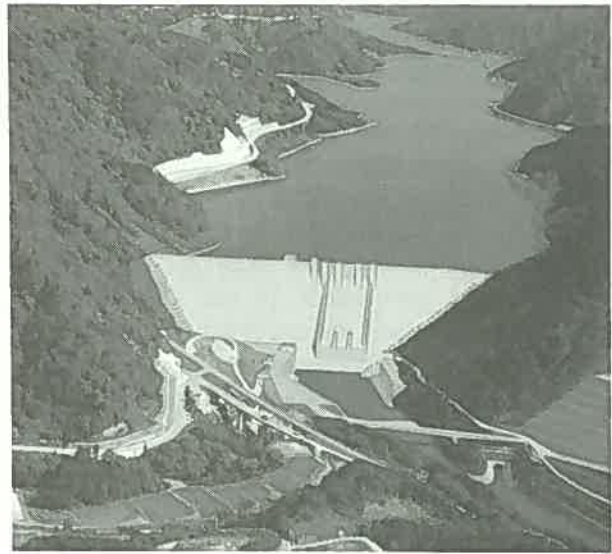
Photo.2 Gassan Dam at Completion
