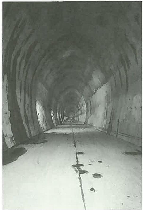
Photo.1 Storage Cavern Excavated Completely
